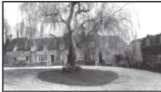
The Stables, Old Leicester Road, today and before conversion
